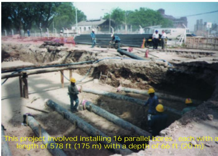
This project involved installing 16 parallel bores, each with a length of 578 ft (175 m) with a depth of 66 ft (20 m).
