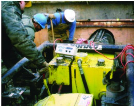
The DigiTrak system provides the operator with real-time pitch and roll position, which aids in keeping the bore on target.
