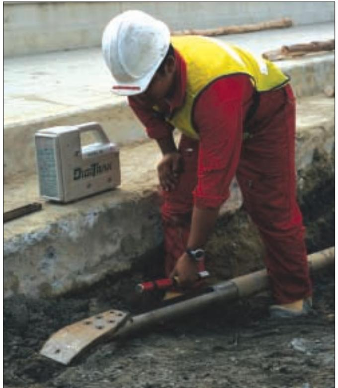
The transmitter is commonly referred to as a sonde, beacon or probe. It is most often battery powered and transmits a magnetic signal from inside the drill tool.
