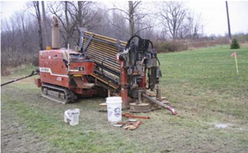
Figure 3. The drill ready to launch the pilot bore
