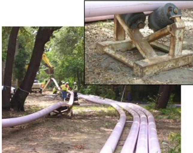
Figure 2. Fusible PVC™ Pipe on Rollers
