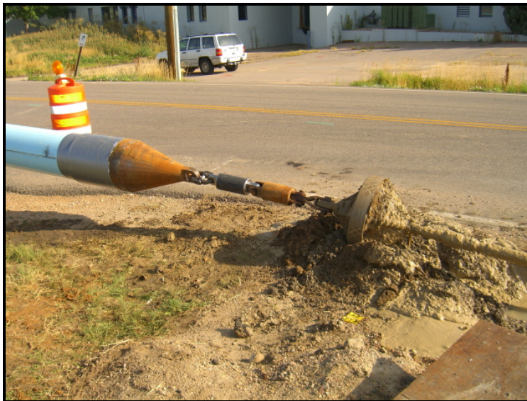
Figure 9. TensiTrak™ In-line Pull Force Measuring Device
